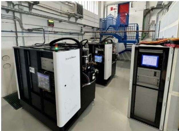
Figure 2: The new X-band and C-band high average power RF sources integrated in the TEX modulator area.
